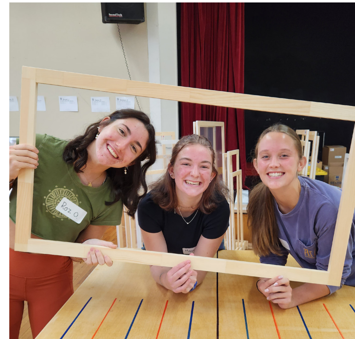
Building window inserts for weatherization at the 2023 Town of Orono Community Window Insert Build • Photo by Dan Dixon
